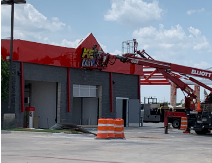
It's exciting to see the sign going up for the Car Wash next to store 317.
