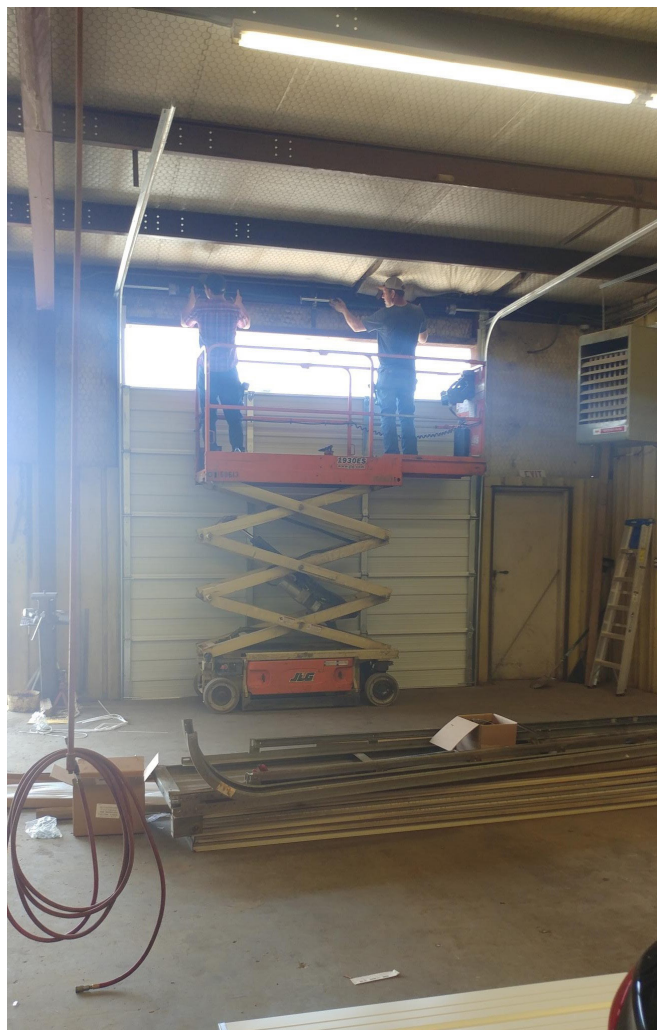
Kent Tire 118 upgrading doors.
