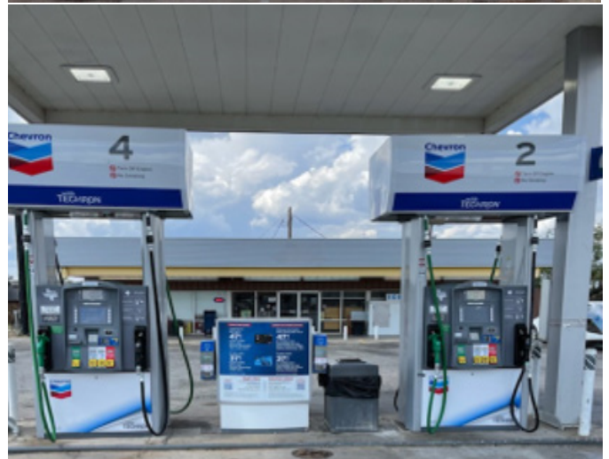
Store 468 in Mineral Wells got the new fuel dispensers this week. Check out the before and after!
