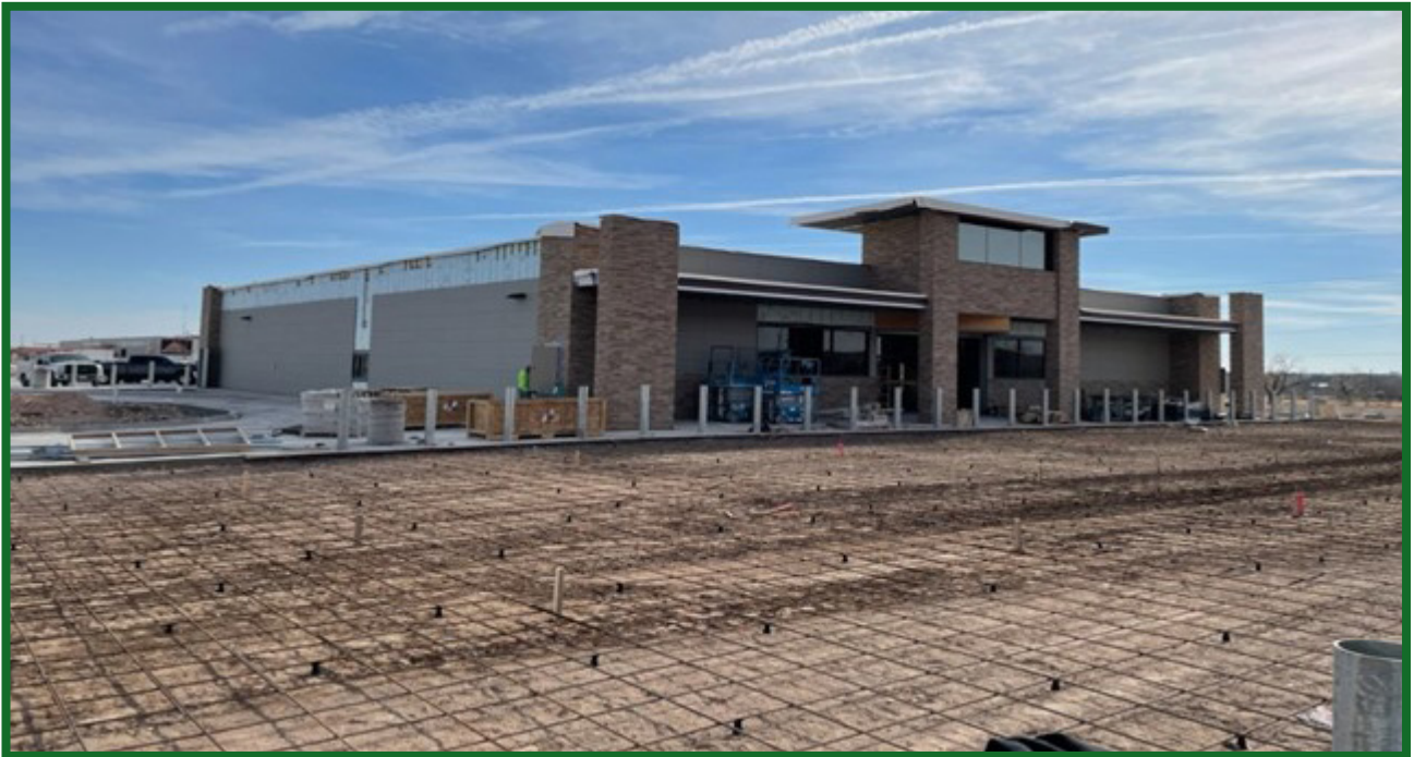
433 Kent Kwik: Paving almost done!
