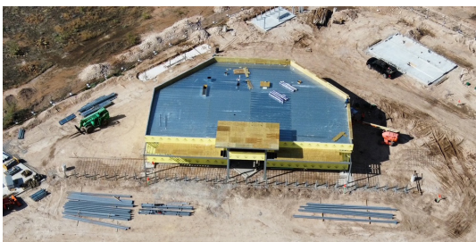
Construction on store 322 is moving along smoothly. The building is up and wrapped; working on interior insulation and utilities!
