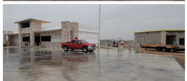
The canopy is up and the building is coming along nicely at store 322.
