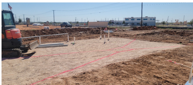
We've gout our building pad prepped and will be pouring the building slab soon for store 326!
