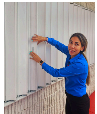
Carla, at 962, checking hurricane shutters, ensuring they are ready for the season.
