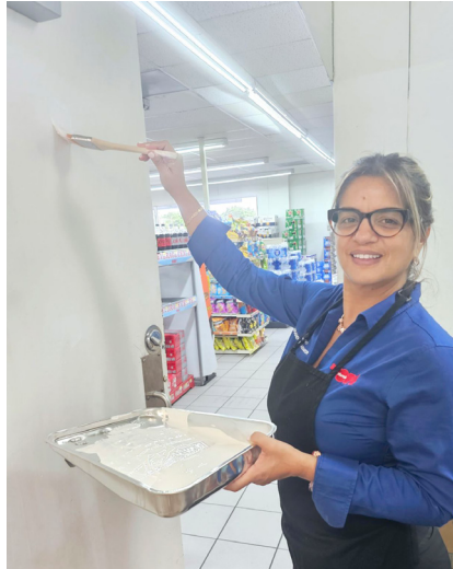
Kathy, manager at 963, touching up the restroom doors to elevate the Guest experience.
