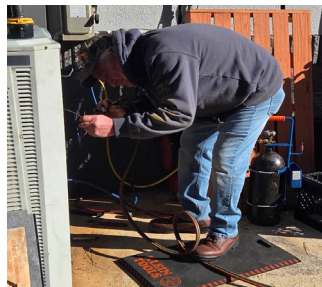
Tim with Maintenance got the heat back up and running on a 29-degree morning. Thank you for jumping in and getting it done!
